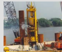
↑ Container-Terminal Altenwerder, Hamburg.
